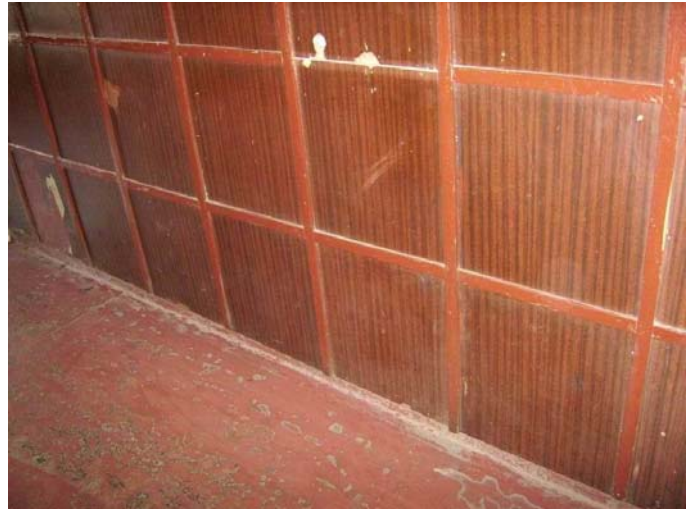
Floor and walls in corridor
