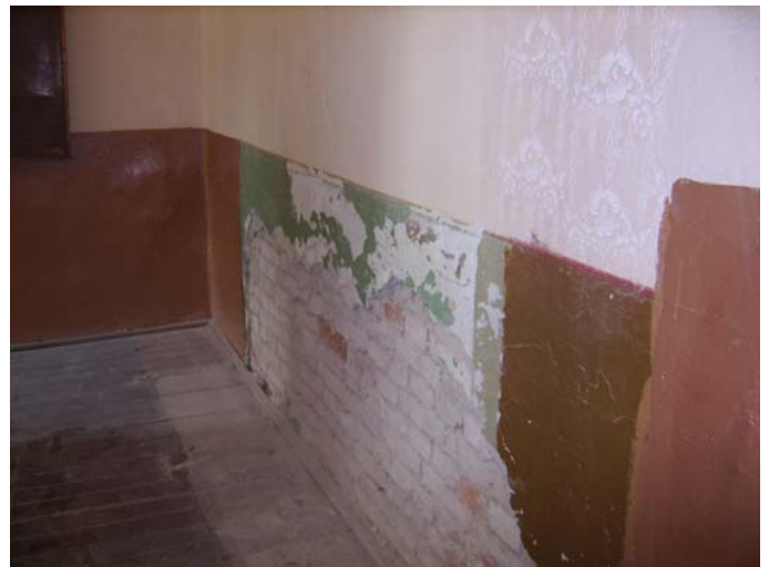
Walls in one of the classrooms
